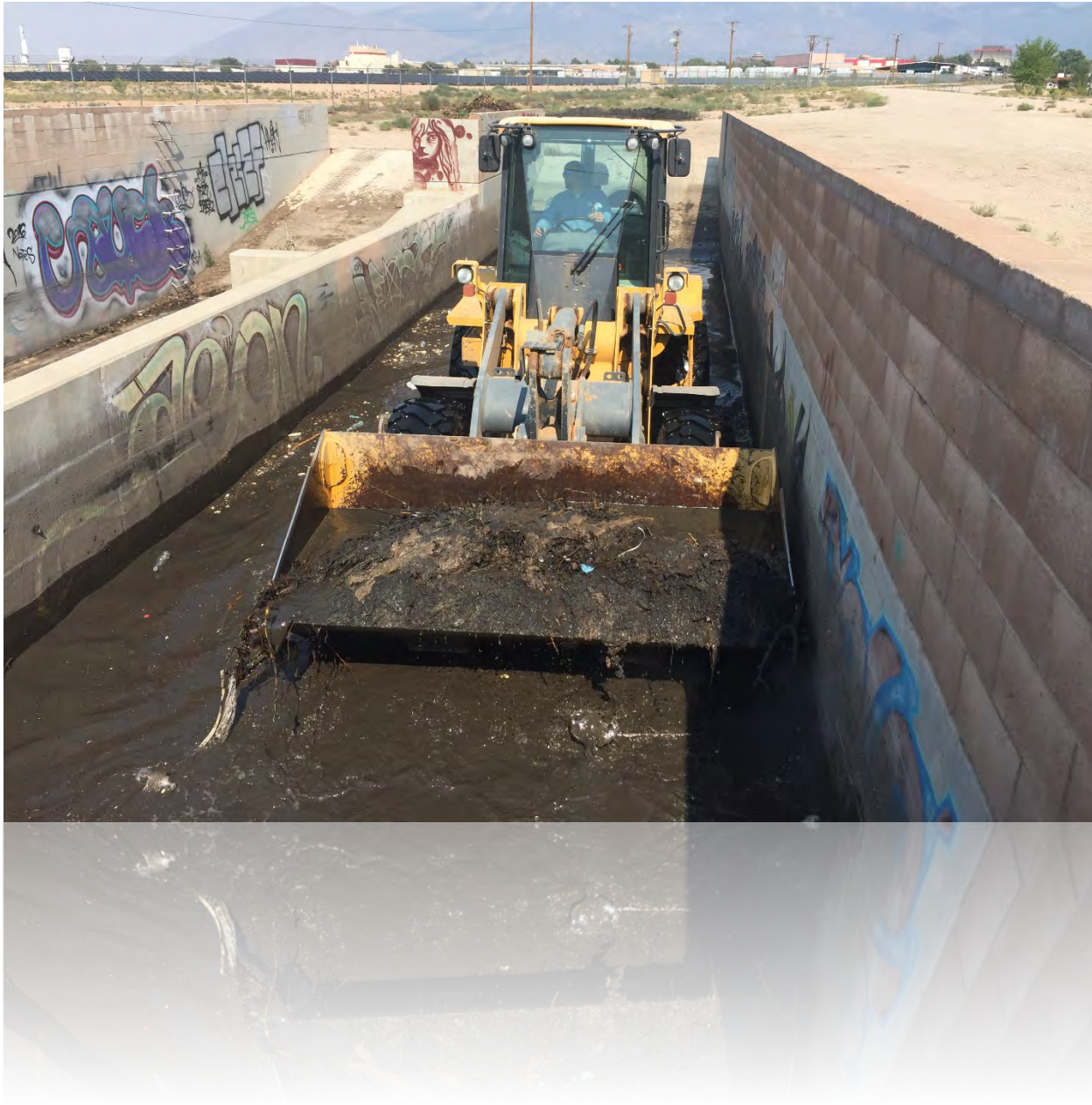
Clean-out activities at a stormwater quality structure
