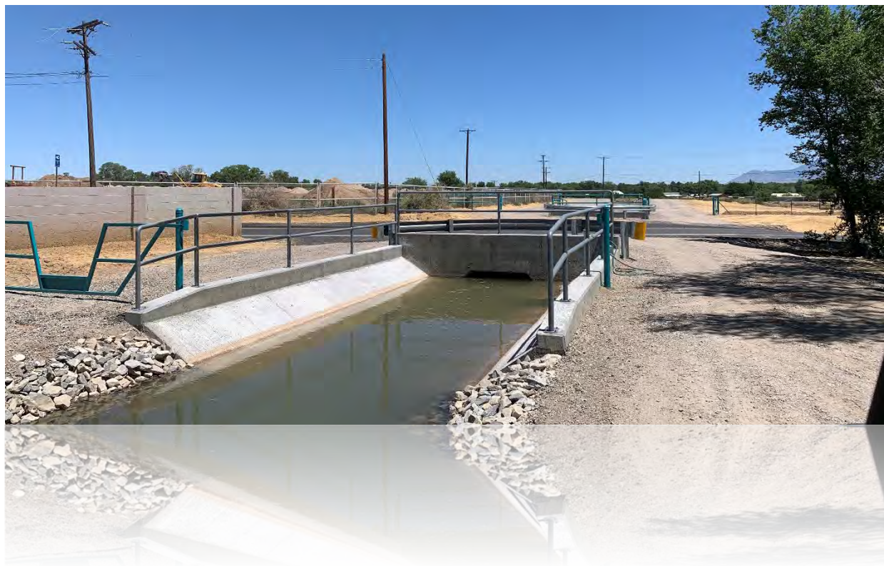
Black Mesa Arroyo: Powers Way crossing, before and after
