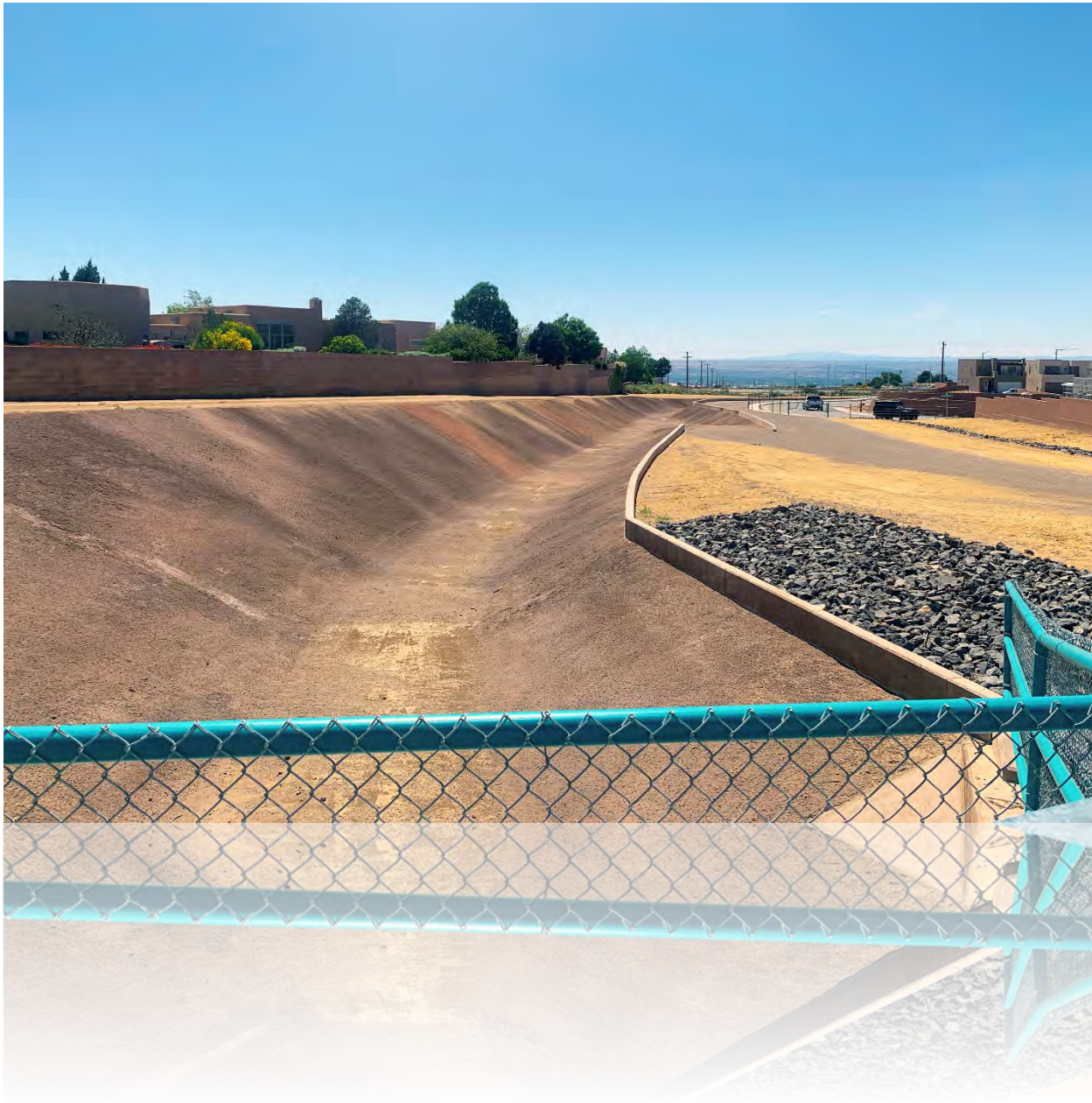
Hawk's Landing on the South Domingo Baca Diversion Channel
