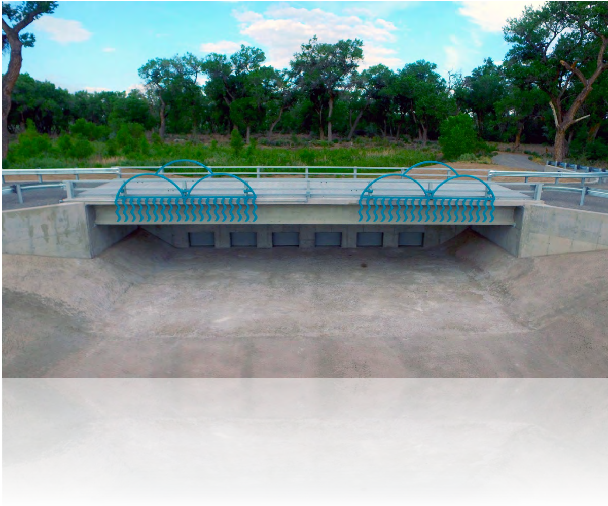
AMAFCA rainclouds enhance the aesthetics of the bridge at the Valle de Oro outlet structure
