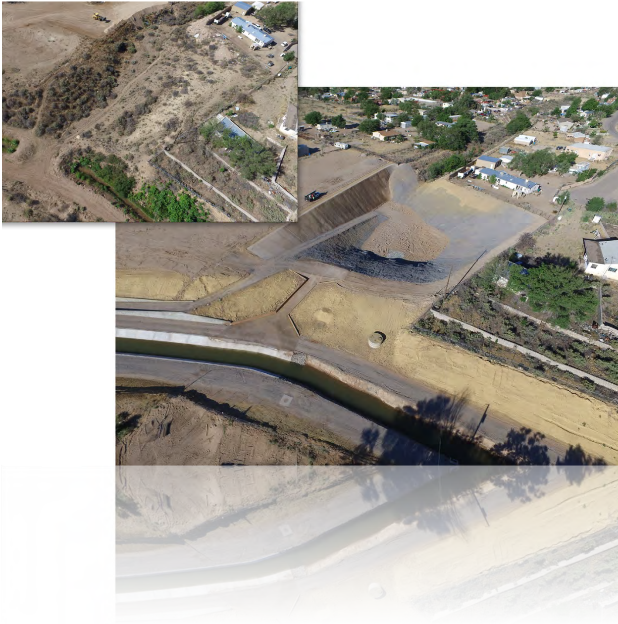
New pond constructed as part of the Black Mesa Arroyo Phase IV Project
