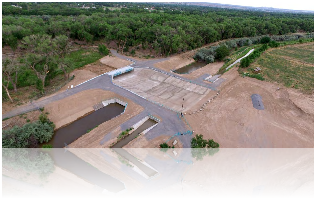
Valle de Oro Arroyo's new crossing facility: conceptual rendering and aerial as-constructed
